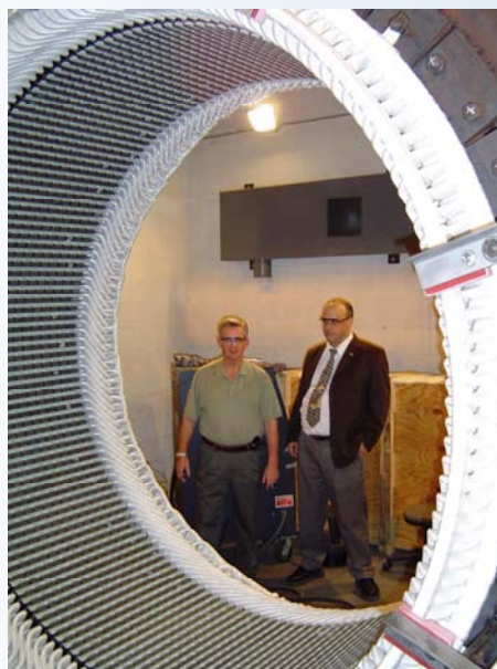
3-D Service chief engineer and VA Tech project manager inspect completed winding.
